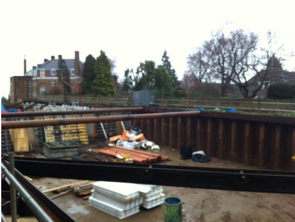
Basement area as excavated including extended area
